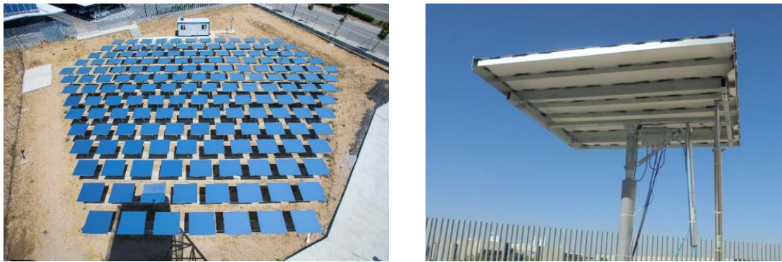
Figure 2: Left: Aerial view of the heliostat field from the top of the solar tower. Right: Lateral view of a 3 m 2 heliostat with two rectilinear actuators.
