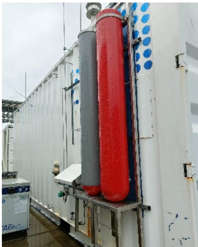
Figure 6: New high-pressure buffer setup with additional HP syngas buffer cylinder of 50L.
