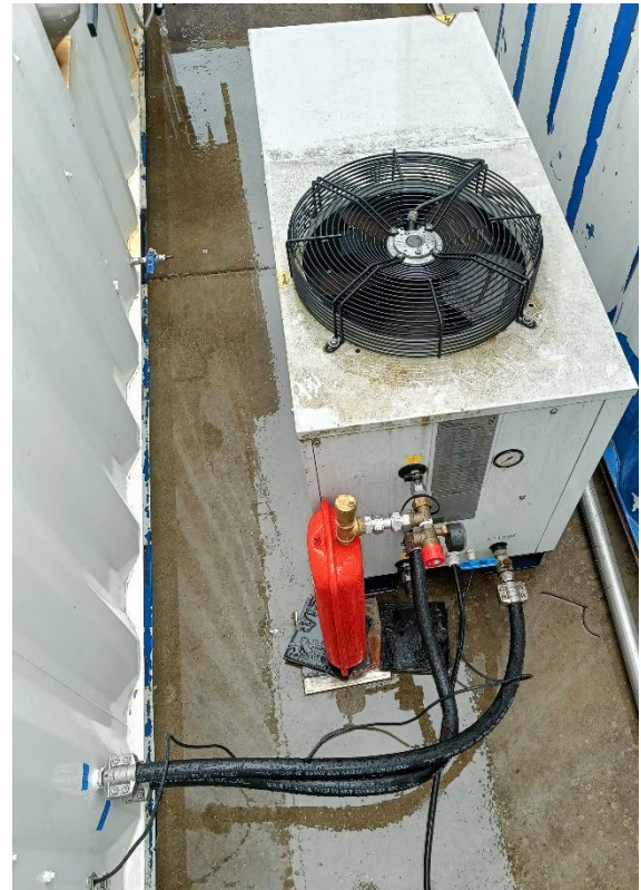
Figure 9: Chiller system with expansion vessel.
